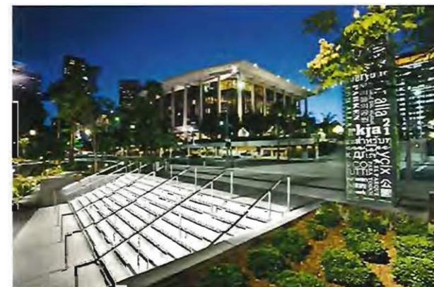
Illuminated steps for safe pedestrian movement
