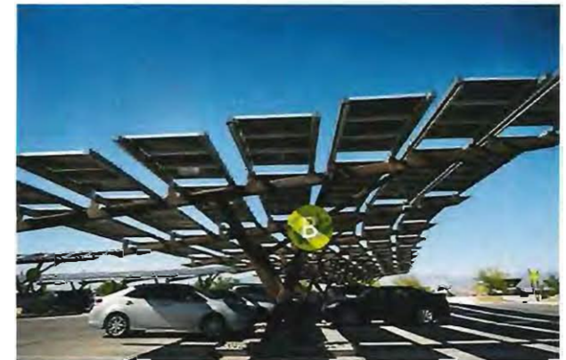
Parking structure with rooftop solar panels
