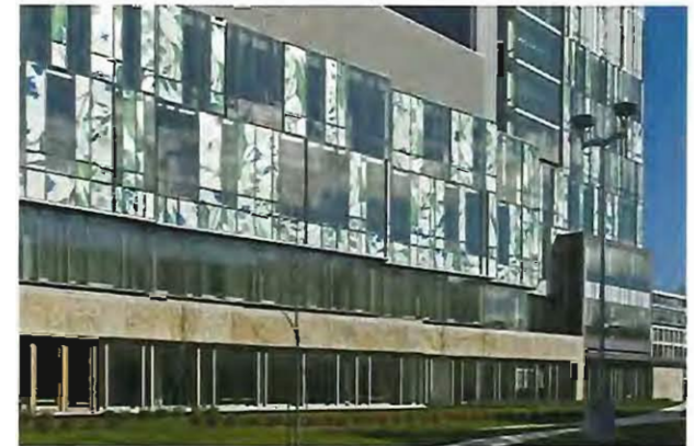
Bird-safe windows through art application at the University of Waterloo
