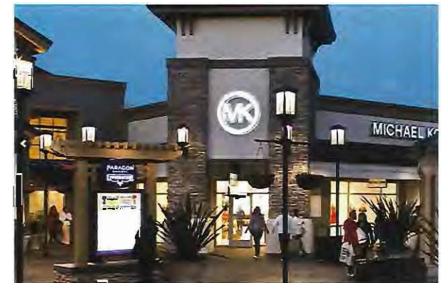
Pedestrian scaled and compatible light fixtures
