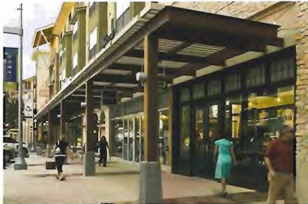
Architectural canopy provides shade and reduces heat gain
