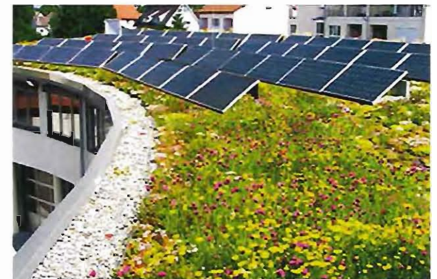
③ Green Roof with Photovoltaics
