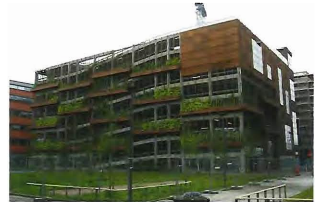
Green parking garage screening
