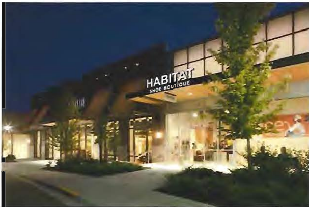
High quality signage that is compatible in scale and character with the building facade
