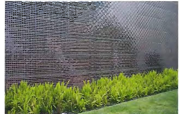
Perforated copper screen keeps birds from colliding with the windows
